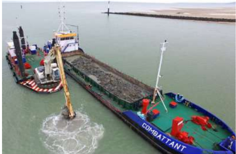
Figure 5 : Example of mechanical dredging (source: Océlian - VCMF)
