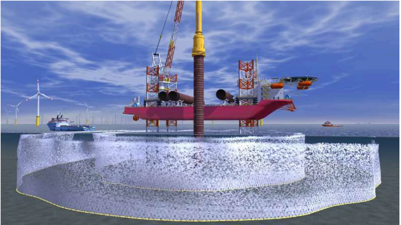
Fig.7. Illustration of the bubble curtain around a pile driving production area (source: Gaia terre- bleue, Impact mer, DHI and Bird&Bird)
