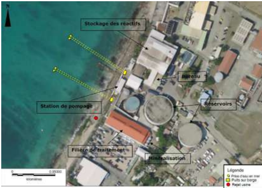
Figure 3 : Aerial view of the plant. Only one of the two pumping lines is operational (source: Safege, 2014).
